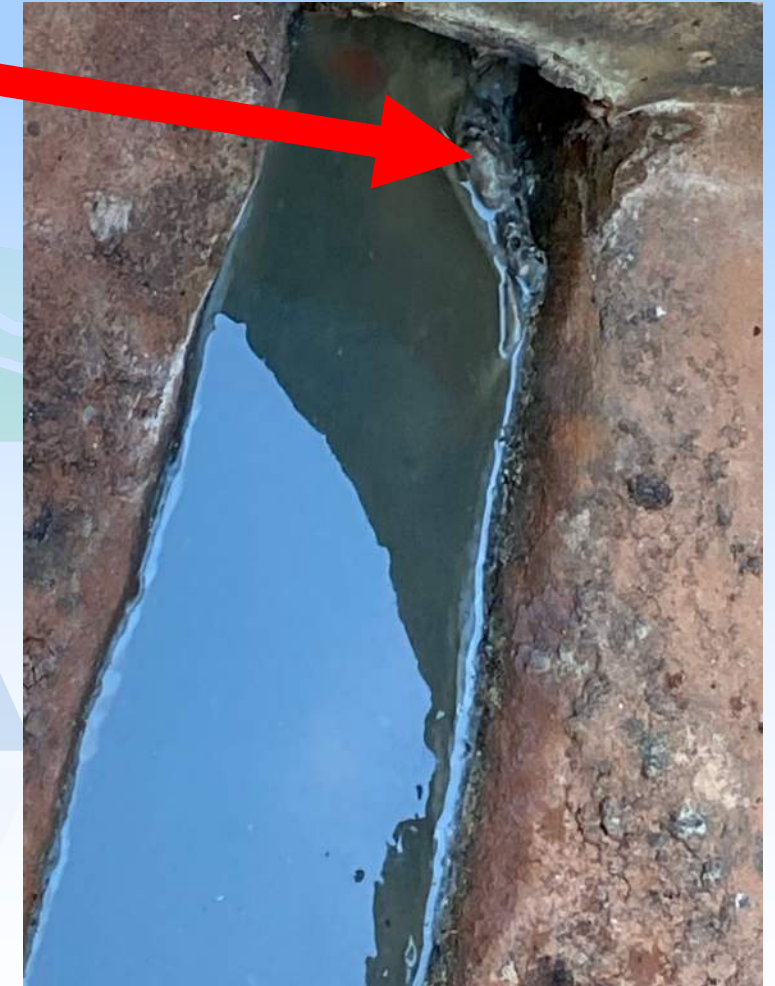
Grease build up on an OJRSA line that was "jetted" from a Member City line into the trunk sewer
