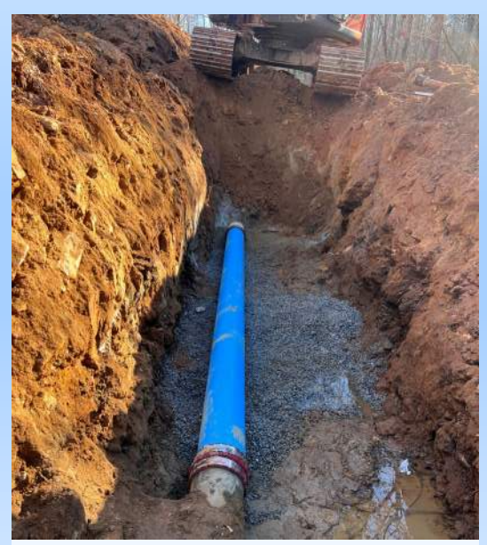
Point repair on broken line
