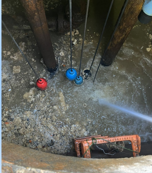
Choestoea PS wet well before cleanout...
