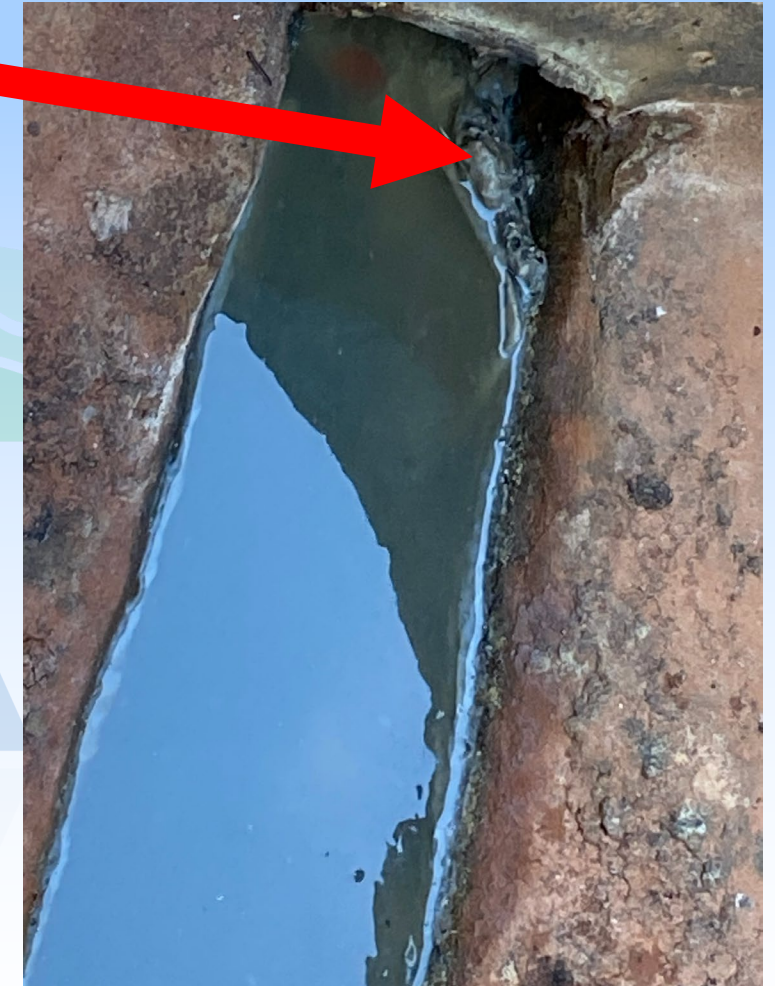
Grease build up on an OJRSA line that was "jetted" from a Member City line into the OJRSA trunk sewer
