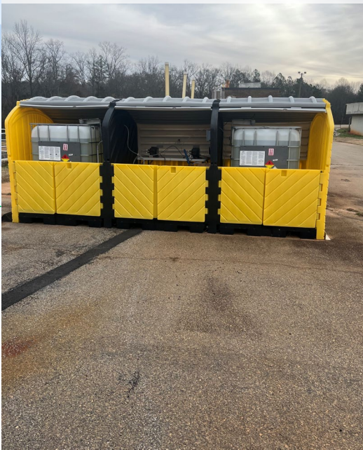
Peracetic acid disinfection system
