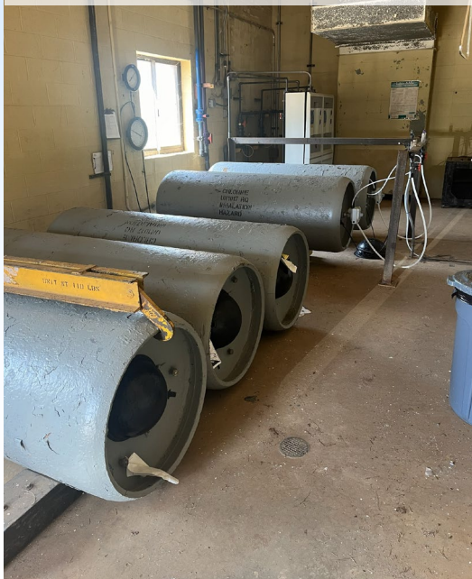
Chlorine gas disinfection system
