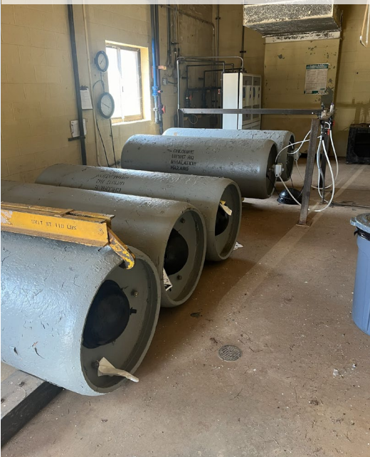
Chlorine gas disinfection system
