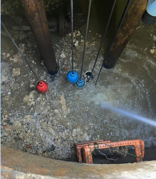
Choestoea PS wet well before cleanout...
