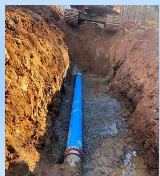
Point repair on broken line
