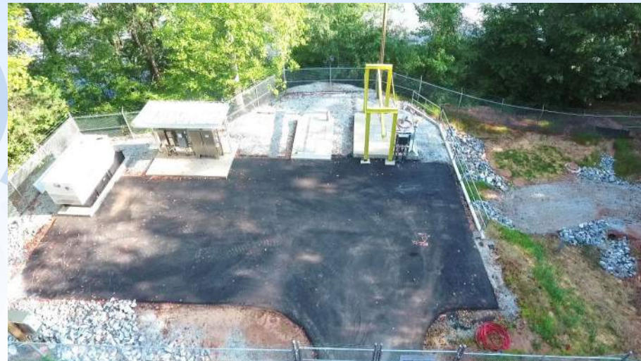
New Duck Pond Pump Station (replacement of Flat Rock PS)
