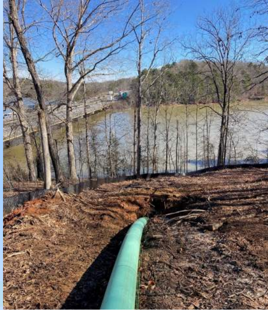
I-85 Sewer Phase II: Pulling force main pipe beneath lake
